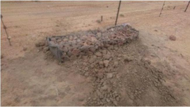
Erosion control work was done on the southern boundary of the estate. Ground was prepared and gabion baskets were built, installed and filled with rocks.
